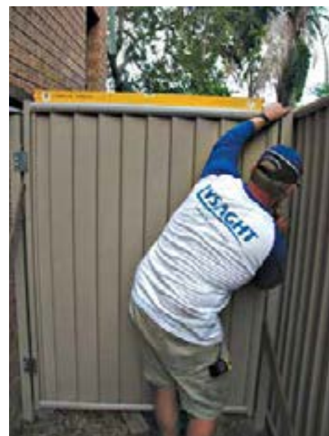
Figure 19.1 Fixing of hinges
