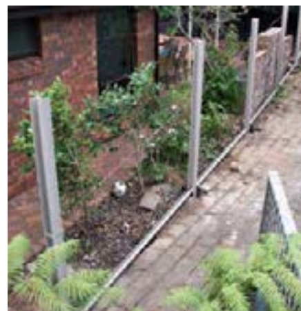
Set all the bottom rails into position ensuring a 50mm ground clearance.
